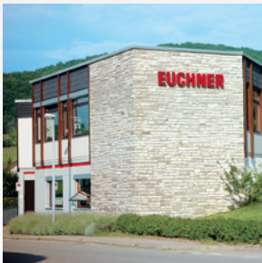
Production location in Unterböhringen
